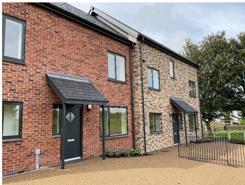
New Council-built homes in Newtown
